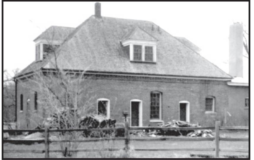
Dairy before restoration
