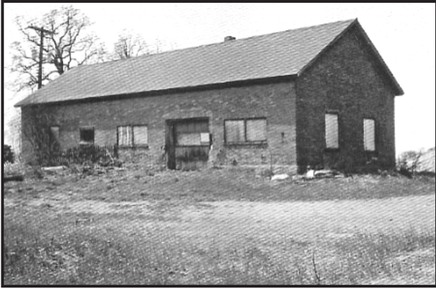
Blacksmith-Machine Shop before restoration
